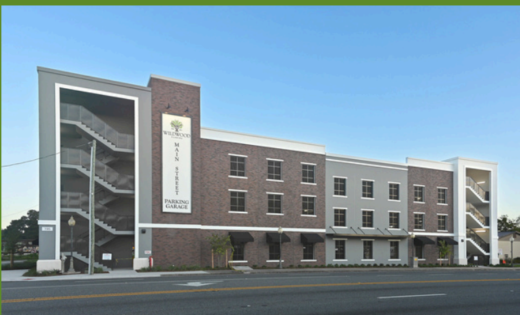
From top: breaking ground in January, construction in progress, and the garage ready to open.
